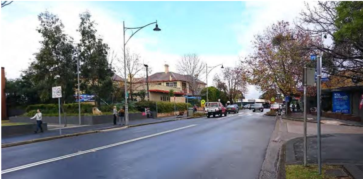
Figure 1-4 - Macquarie Road looking west
