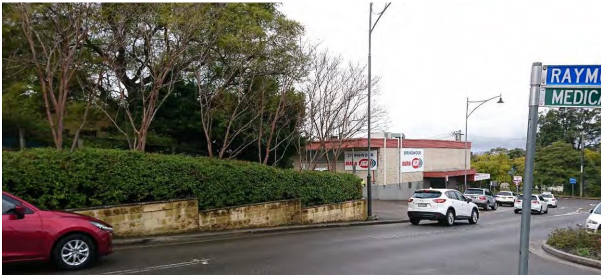
Figure 1-7 - Raymond Road frontage - former IGA
