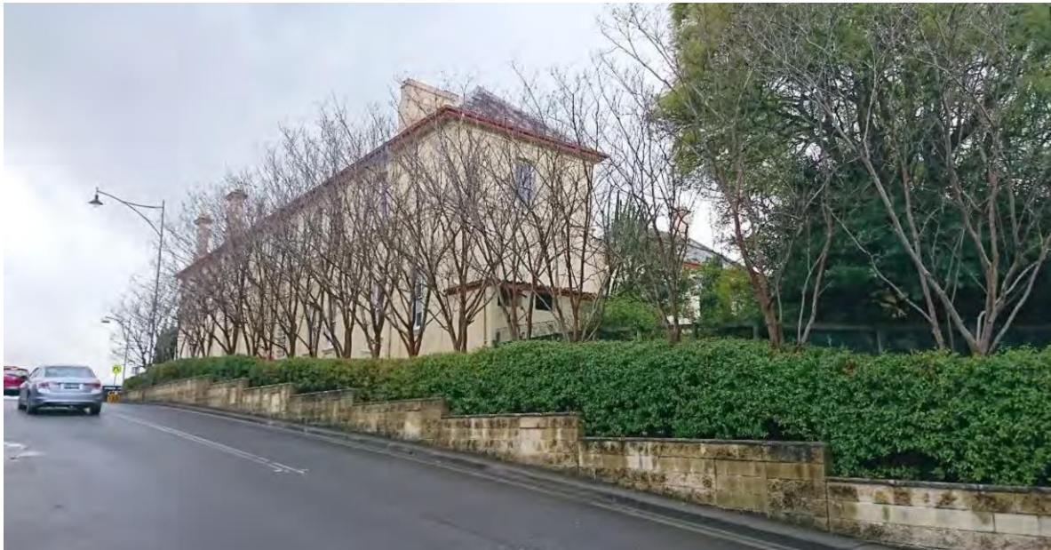
Figure 1-6 - Raymond Road frontage - Oriental Hotel
